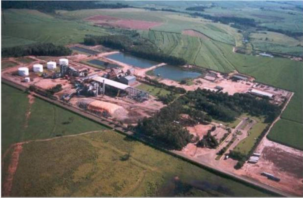
Aerial view of the sugar plant (source: Unialco S.A.)
