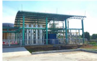
Purification Facilities(biogas 160m 3 /h) and NGV station at the ABC palm mil in Nakhon Si Thammarat
