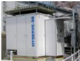
H 2 production equipment(30m 3 /h) in Motomachi factory of Toyota, Japan
