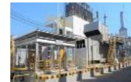
On-site cogeneration(7MW) plant in Thailand
