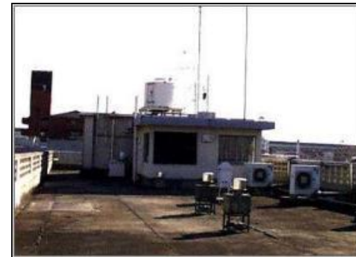
Air Pollution Monitoring Station
