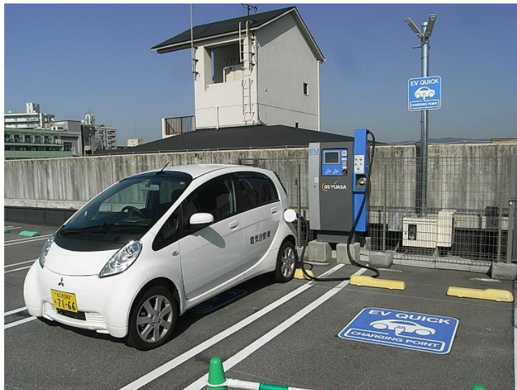
Electric Vehicle Charging Station
