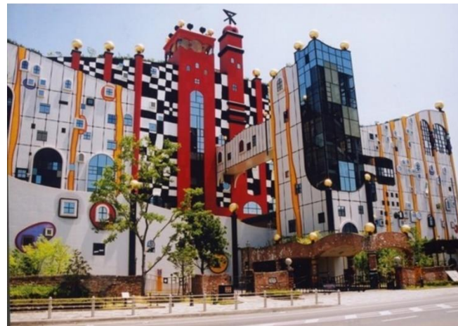
Maishima Incineration Plant, Konohana Ward, Osaka City
