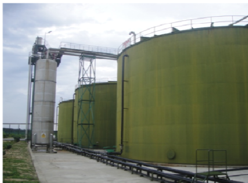
Sungei Kahang POME Biogas Project in Kahang, Johor, INDONESIA
