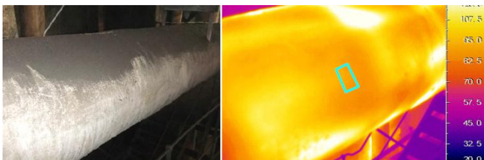
Figure AP2-1.1 Example of thermographic image pixels extracted for only area attached by the heat flow sensor without installation of project thermal insulation material
