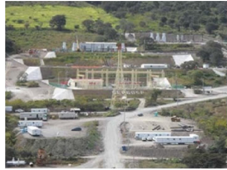
Geothermal power generation, Mitsubishi Hitachi Power Systems, Mexico
