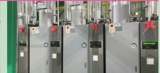
Once-through Boiler (Indonesia) DIC Corporation
