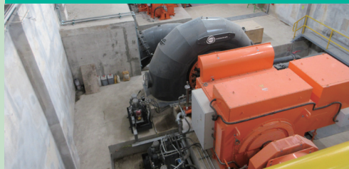
Mini Hydro Power Plant (Indonesia) WWS-JAPAN Co.
