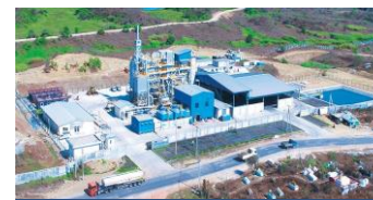
Waste to Energy Plant, JFE engineering, Myanmar
