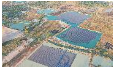
Floating Solar PV, TSB Co., Ltd., Thailand
