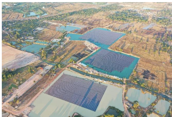
Floating Solar PV, TSB Co., Ltd., Thailand
