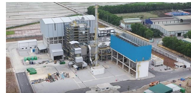
Waste to Energy Plant (Vietnam) JFE Engineering Corporation
