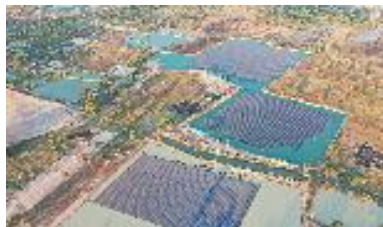
Floating Solar PV, TSB Co., Ltd., Thailand
