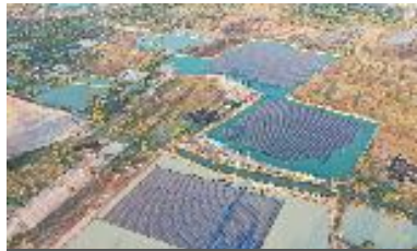
Floating Solar PV, TSB Co., Ltd., Thailand
