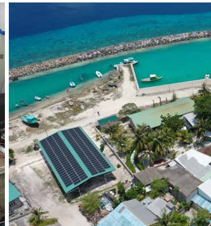
Solar PV at the project site
