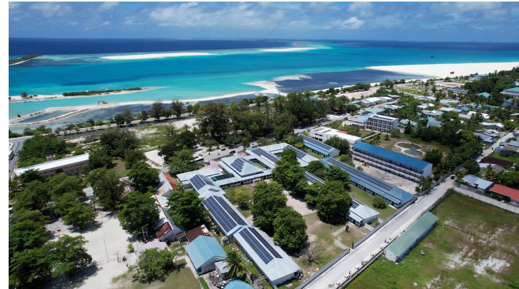
Renewable Energy Installation in Maldives
