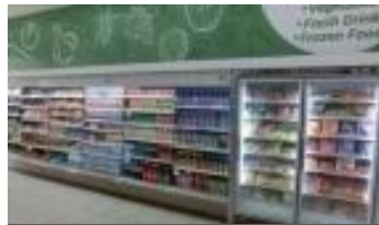
Energy saving at convenience stores, Panasonic, Indonesia
