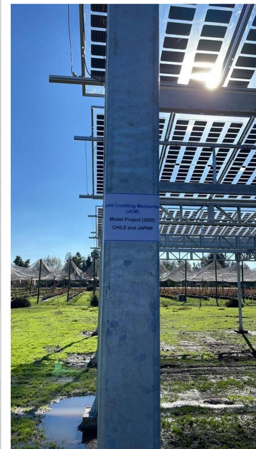
Solar Farm Panels with transparent backsheet of 54% transmittance
