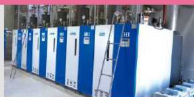
Once-through Boiler(Myanmar)/ Acecook Co., Ltd.
