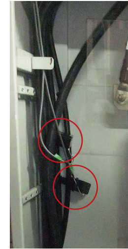
Current sensor installation
