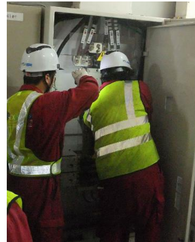
Current sensor installation
