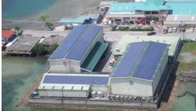
Small Scale Solar Power Plants for Commercial Facilities in Island States (Palau)
