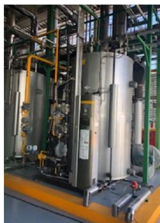
JCM Model Project (2016) [have been started operation] Introduction of Once-through Boiler and Fuel Switching to Tequila Plant
