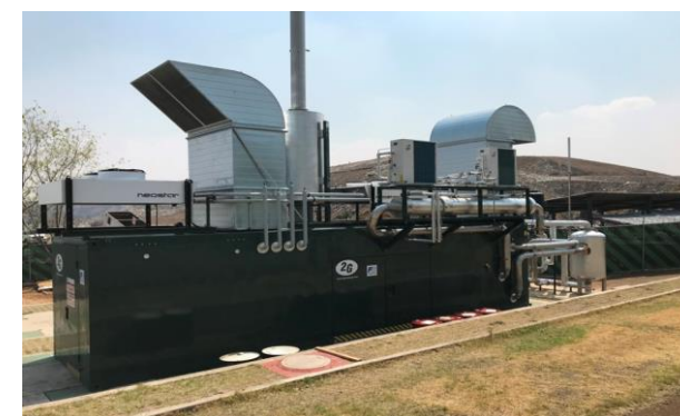
JCM Model Project (2016) [have been started operation] Introduction of 1.2MW Power Generation with Methane Gas Recovery System
