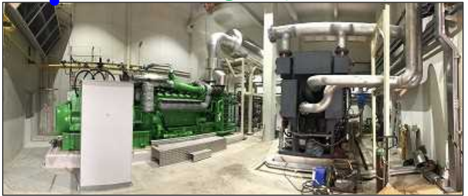
Gas Engine (+Chiller) Room
