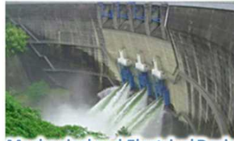
Mechanical and Electrical Design MEP Planning and Design for Large-Scale Infrastructure and facilities, etc.
