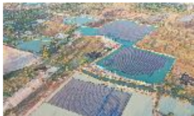
Floating Solar PV, TSB Co., Ltd., Thailand
