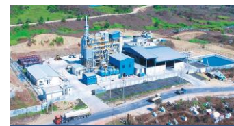
Waste to Energy Plant, JFE engineering, Myanmar
