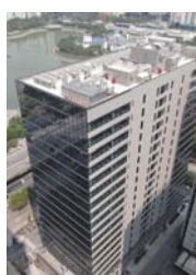
No.21-2: Demonstration project of the stylish and high-efficiency BIPV system to the high-rise building in Thailand
