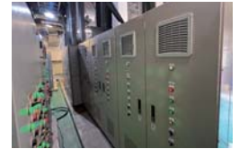
No.20-3 Load-linked flow control system
