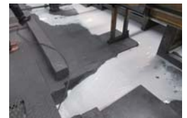
Survey on wastewater including oil from factory
