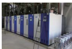
No. 17: Introduction of High-efficiency Once-through Boiler in Instant Noodle Factory (installed boilers)
