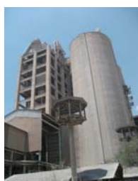
Utilising exhaust heat at a cement manufacturing plant (Indonesia)
