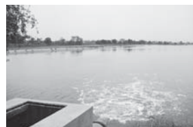
Stabilization pond (outlet to 1st pond)
