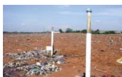
Biogas analysis wells at waste landfill site (Kajima Corp.)
