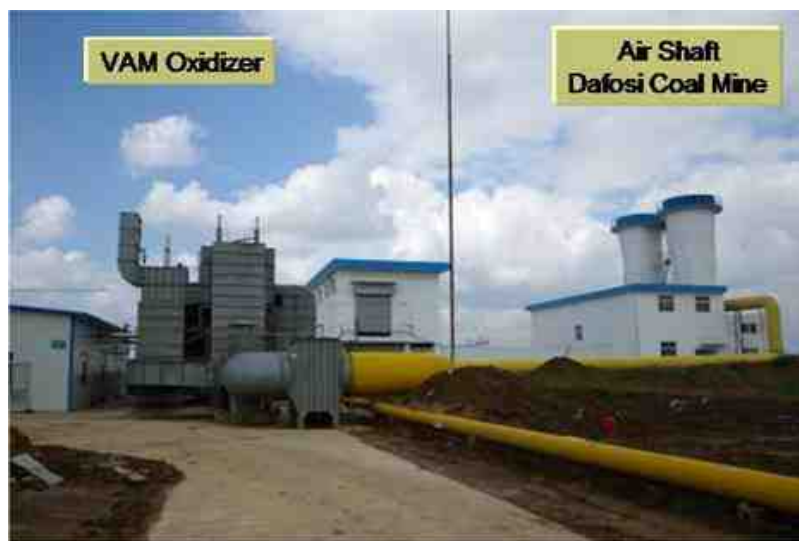
Figure -2 Installation of the VAM Oxidizing System at Dafosi Coal Mine of Binchang Co. for full scale field trial.
