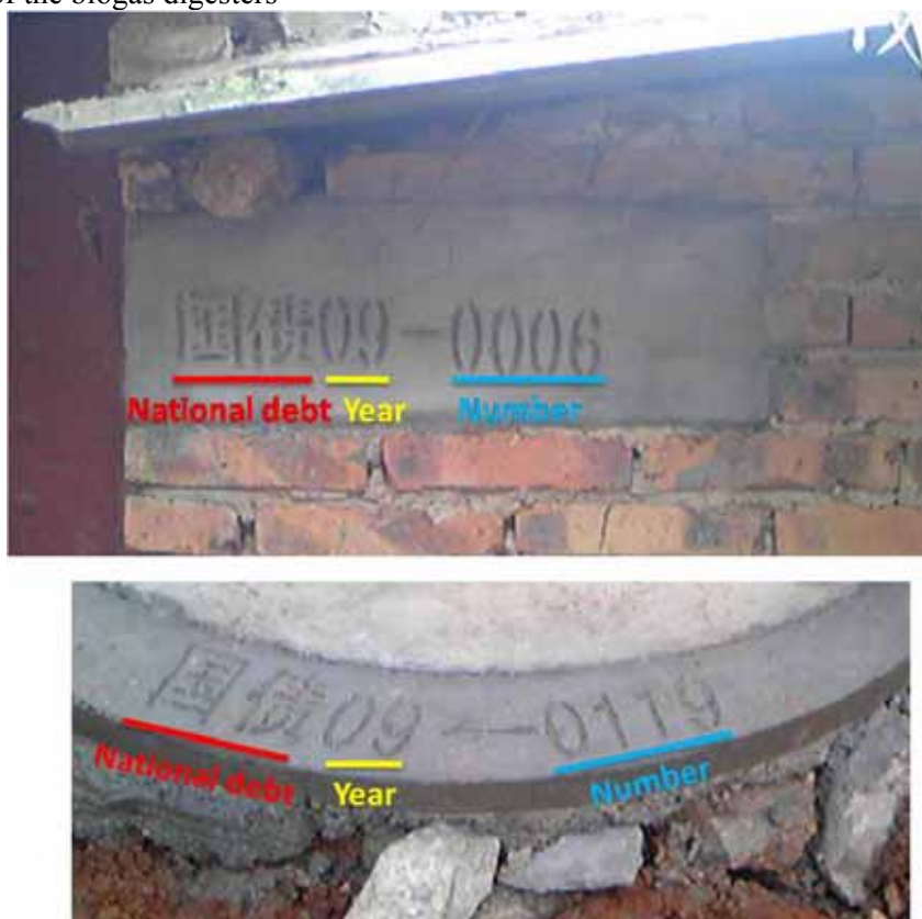
Figure 3 Mark of biogas digesters
