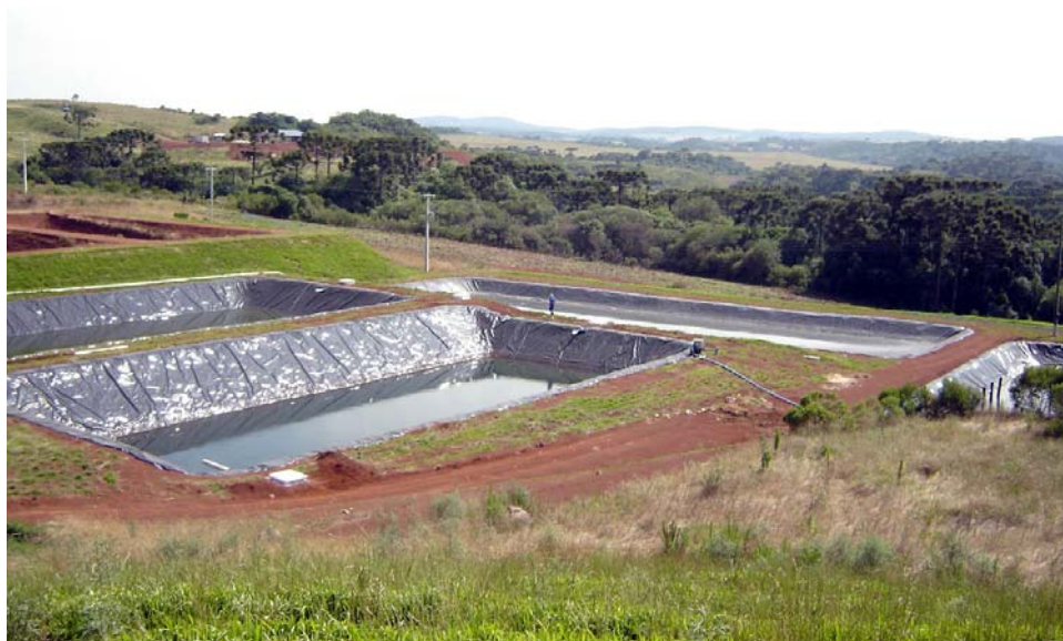
Figure 2 Anaerobic lagoons currently used in the baseline scenario
