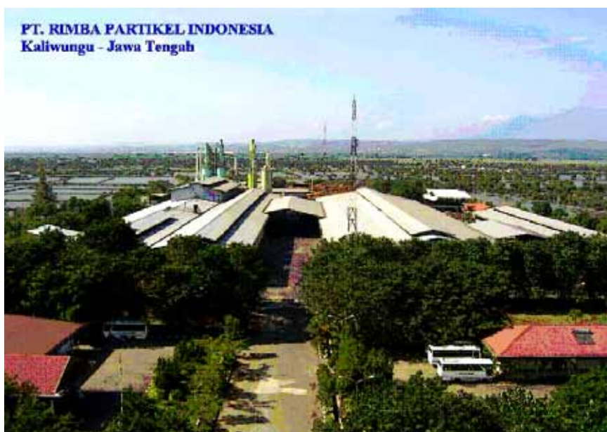
Fig-1: Full view of the plant
