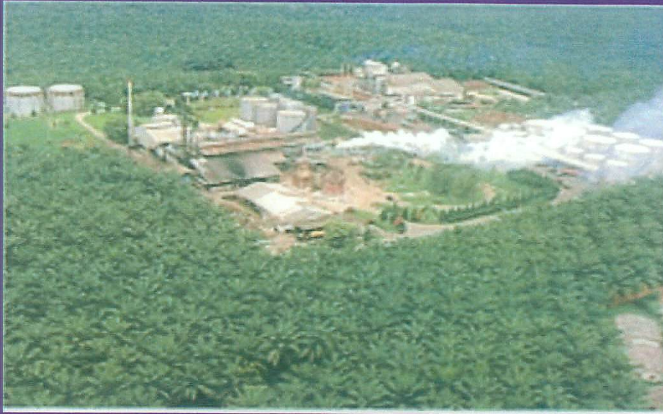
Aerial Photo of Keck Seng (M) Bhd Masai Palm Oil Mill/Refinery
