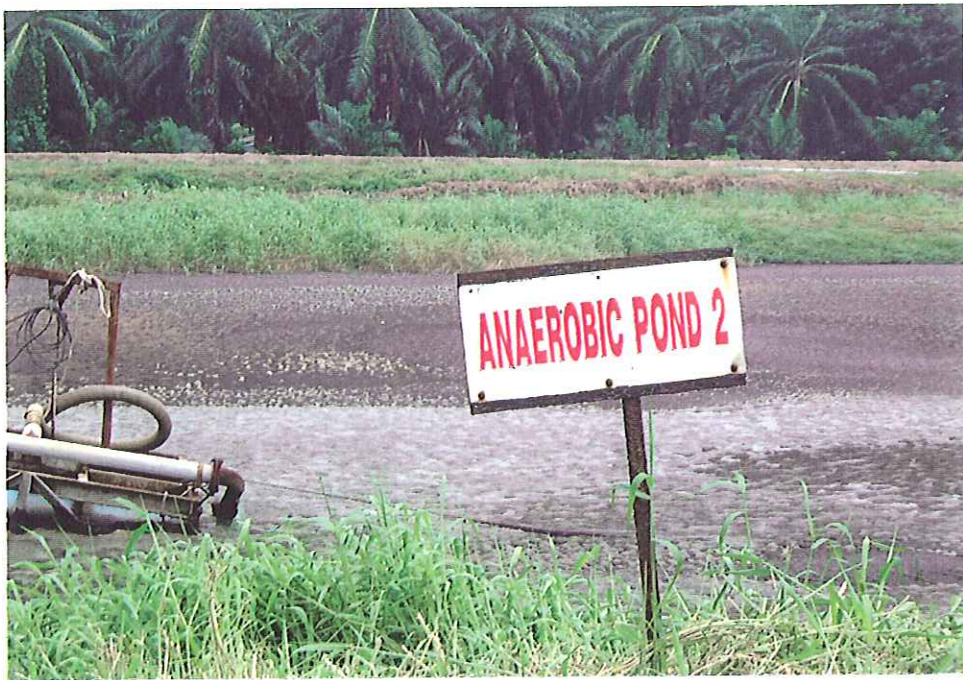
Anaerobic treatment pond (Lagoon)
