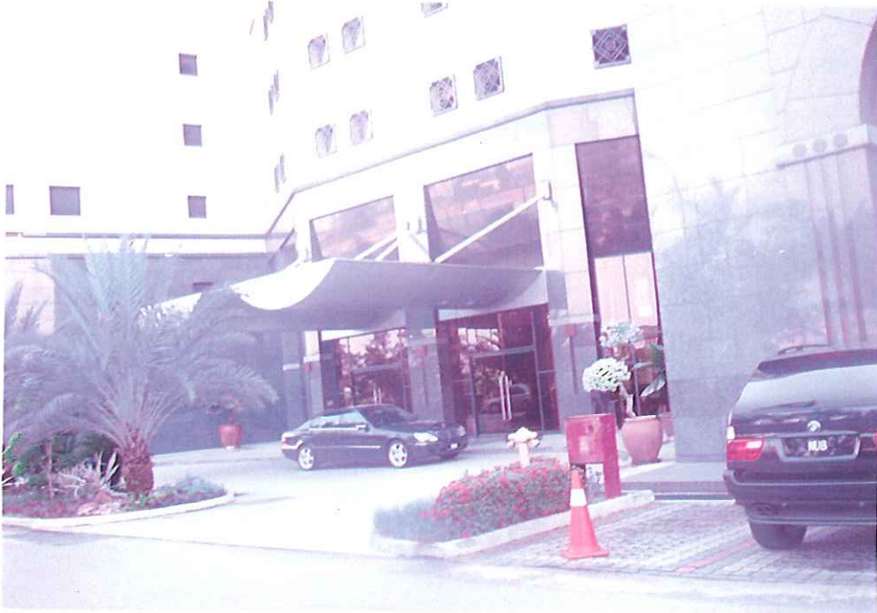
PTM office entrance
