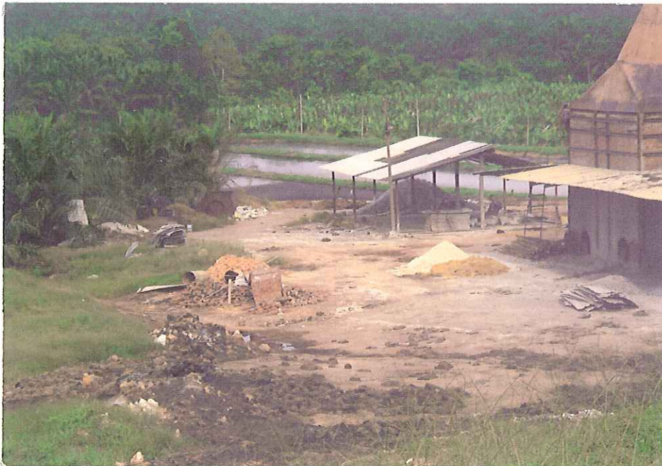
Planning installation site of digesters
