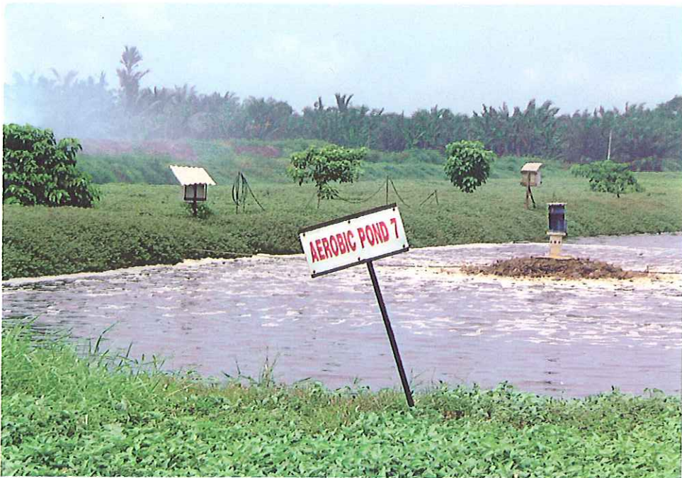
Aerobic treatment pond (Lagoon)
