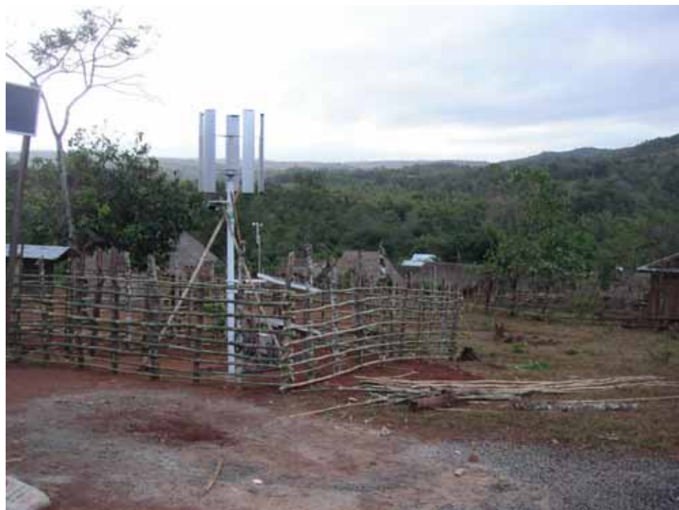
Figure 2. Planned site for the installation of the hybrid power system
