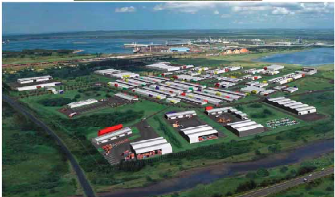
Figure PDD-2: Present Situation and Future Image of the Industrial Zone 1A
