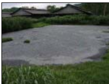
e) Upstream of the anaerobic lagoon. Methane bubbles on the surface.
