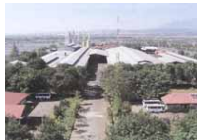
Fig. A-2 Full view of the factory
