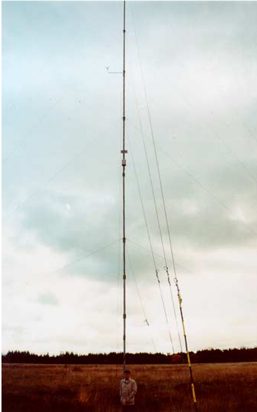
The wind measurement mast in Pakri Peninsula
