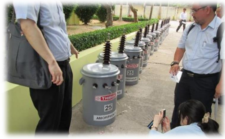
Checking installed AMDTs
