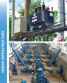
Viet Nam / Yuko Keiso Co., Ltd. Amorphous High Efficiency Transformers in power grid
