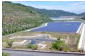
First IPP Plant by SHARP
