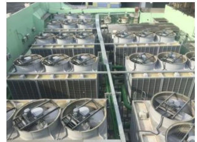
Cooling Towers after replacement
