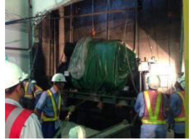
Lifting Chiller from unloading shaft
