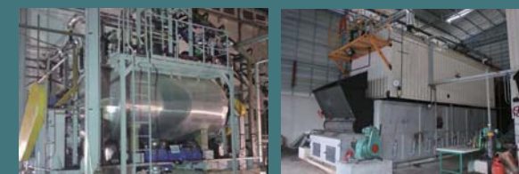
Waste power generation by subcritical water treatment technology (hydrolysis treatment)
