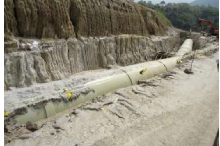
GRP Pipe Installation
