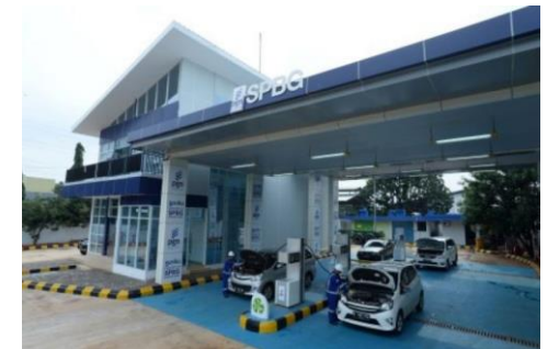
Gas Fuel Station (SPBG)
