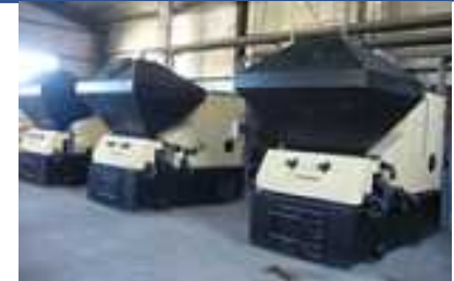
High-efficiency Heat only Boilers, Suuri-Keikaku, Mongolia
