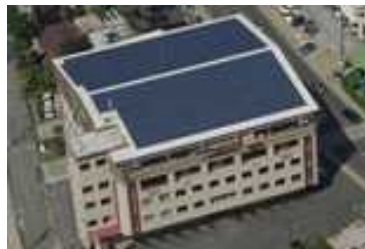
Installing solar PV system, PCKK, Palau Maldives
