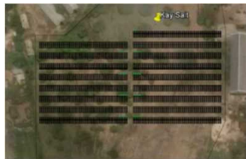
Solar PV System at Salt Factory, PCKK, Kenya
