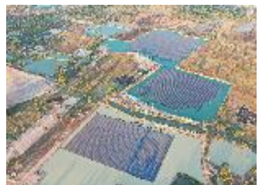
Floating Solar PV, TSB Co., Ltd., Thai
