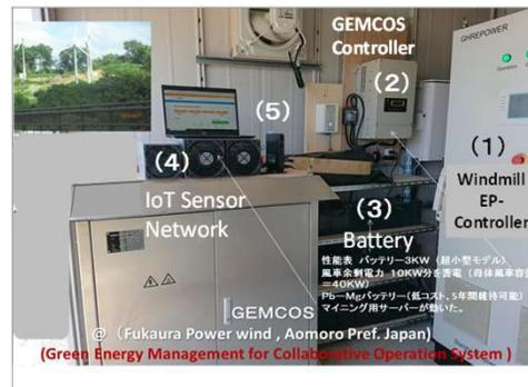
Fig. The control system block diagram using surplus electric power in GEMCOS
