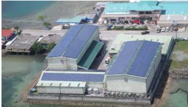
Small Scale Solar Power Plants for Commercial Facilities in Island States (Palau)
